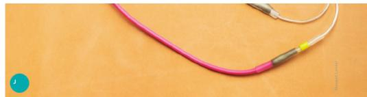
7. Use the heat gun to shrink the tubing until it is snug [Figure
